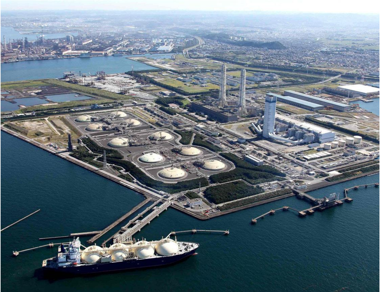
Picture 3-10 Futtsu regasification plant and LNG Terminal (“Japan,” 2012)
