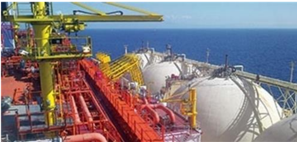
Picture 4-6 STS loading arms (Mike Corkhill, 2013)
