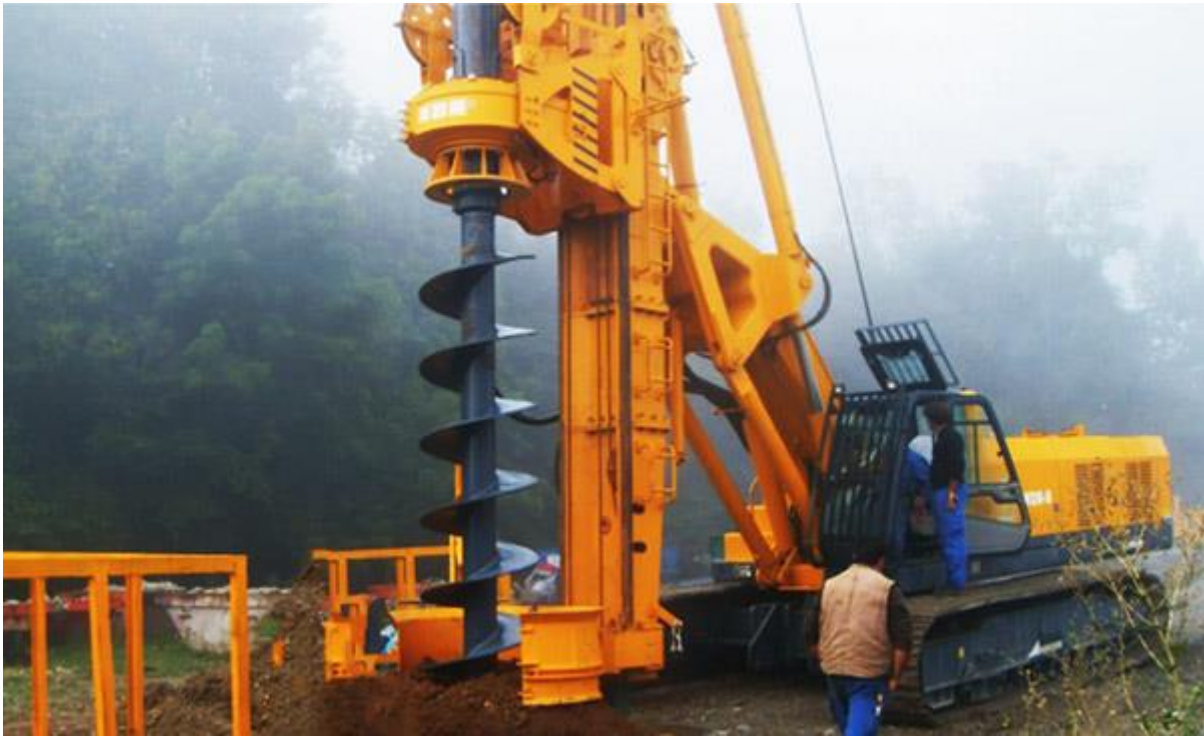
Picture 3-4 Rotary Drilling Rig (“SWDM22B,” 2017)
