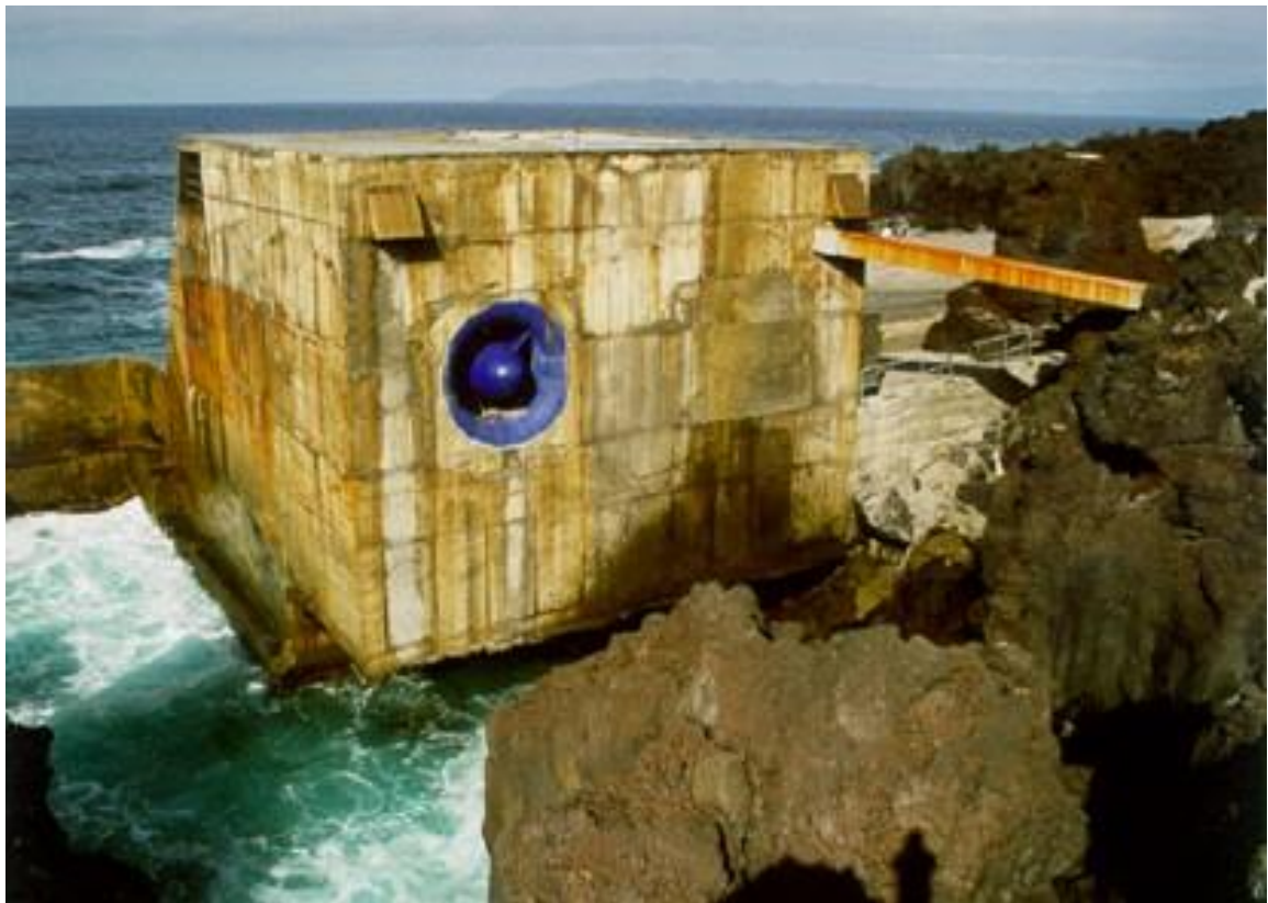
Figure 31. Wave power plant Pico at the Azores [Falcão, 2005]
