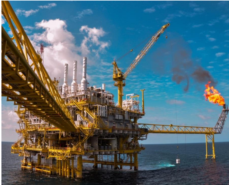
Figure 16. Jacket platform at the gulf of Thailand [ www.dlubal.com ]
