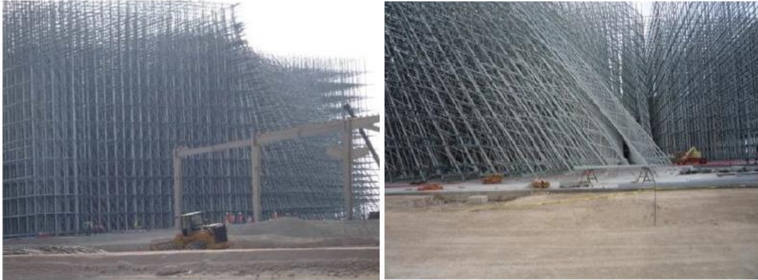
Figure 1.4: Partial collapse of a ARSW during construction phase
