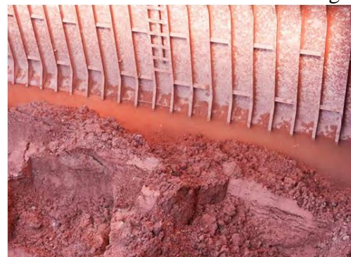
Figure 21 Failure Mechanism of Bauxite cargo (Global Bauxite Working Group, 2017)
