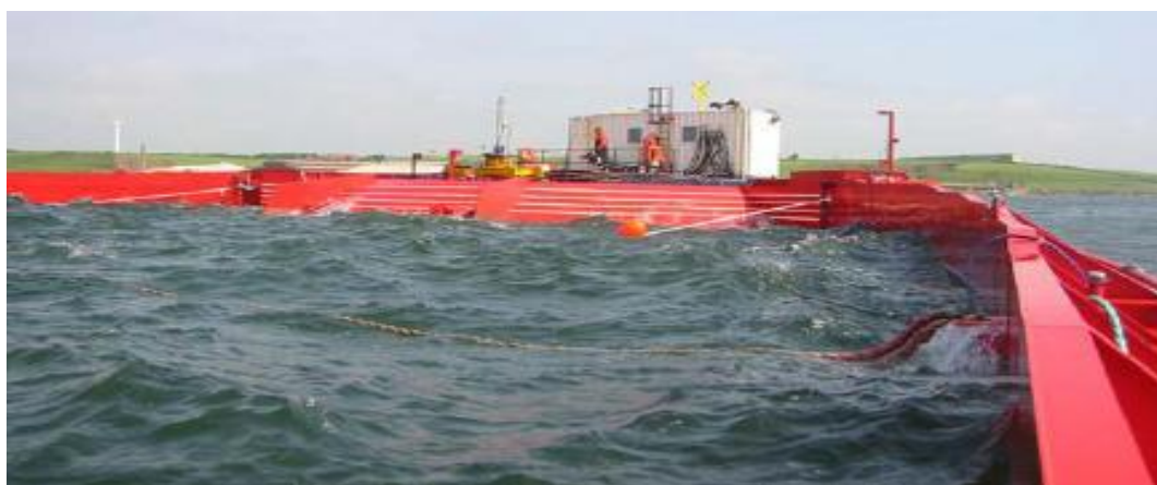
Figure 1.7: Overtopping: the Wave Dragon (Kofoed et al. 2006).
