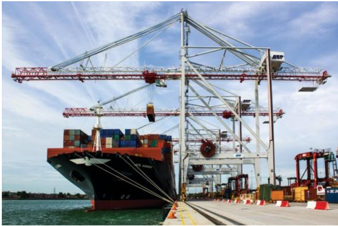
Figure 2. STS cranes operating on a container ship (Liebherr).
