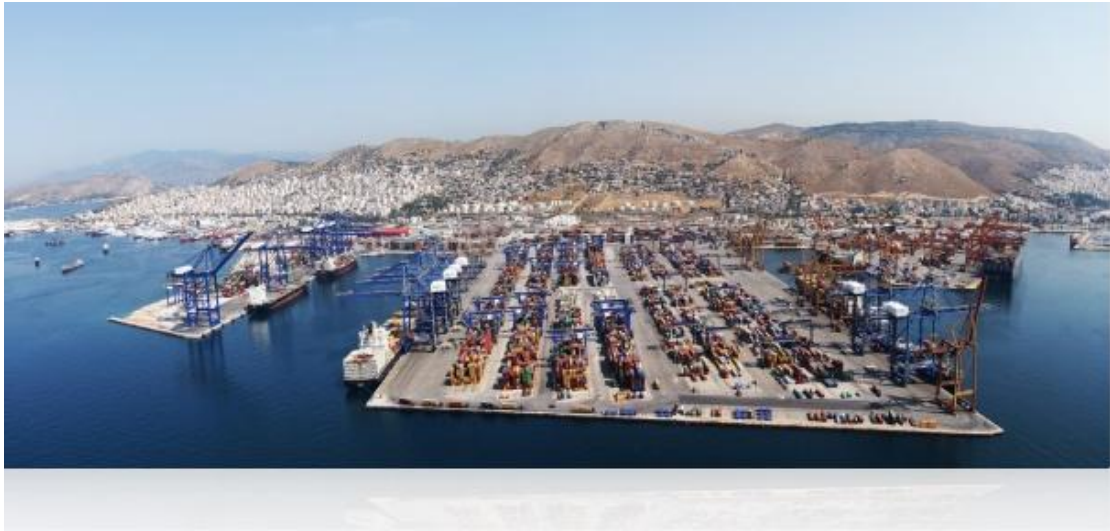
Figure 38. Piraeus Container Terminal (PCT)
