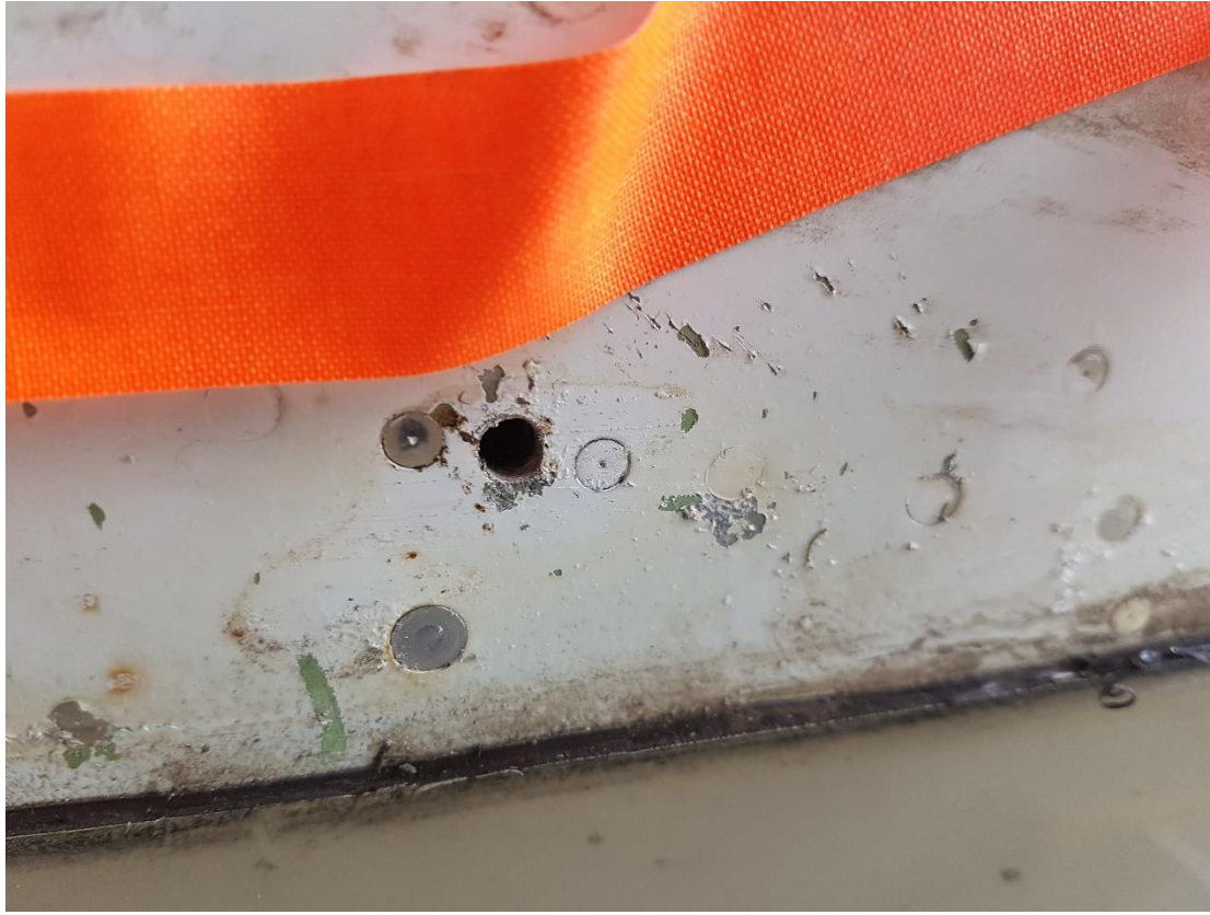
Photo 5.2e: Corrosion in fairing areas
