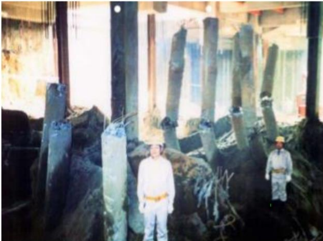
Picture of the piles at the Kobe earthquake 1995 in Japan. One of the first observations of failures at depths that didn't coincide with the dynamic loadings and introduced the kinematic loadings to the world.
