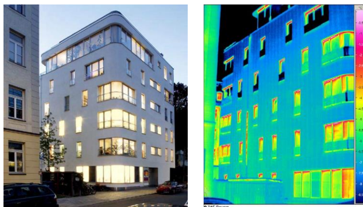
Figure 3.20 – The building in Munich and the thermographic scan [63].
