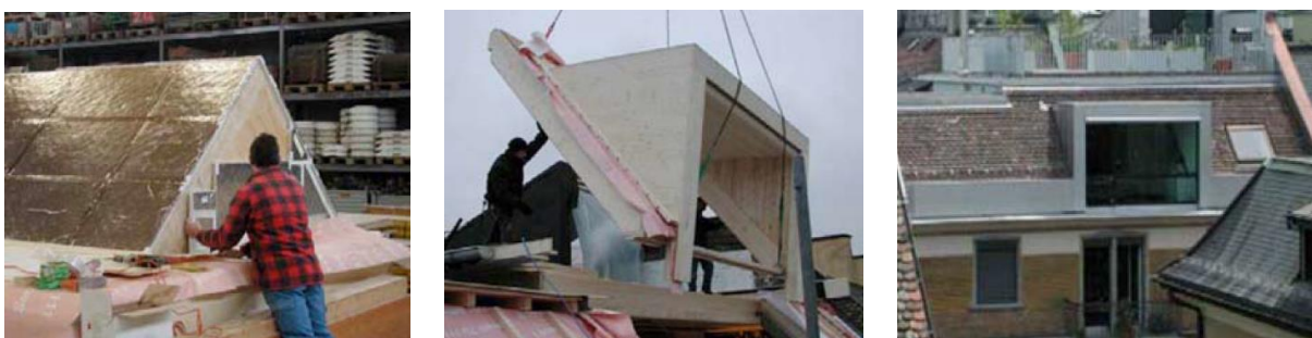
Figure 3.19 - Prefabrication, installation and view of the finished dormer window [57].
