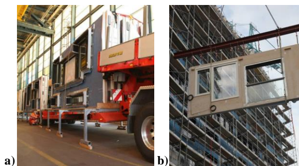
Figure 1.4 – Prefabricated wall assembly: a) transportation and b) final installation [40].
