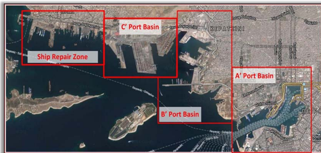
View of PPA's facilities and businesses (Source:: Domosferon, 2018)
