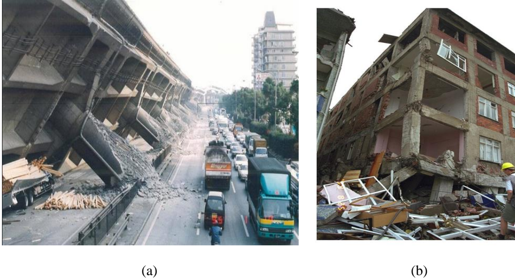
Fig. 1.2 (a) Bridge collapse after the Kobe earthquake in Japan 1995, (b) Failure of beam column exterior joint (Sezen et al. 2000 [2]).
