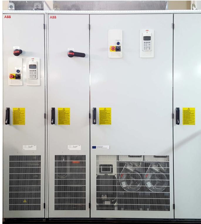
Figure 2.7: ABB ACS 800 controlling panels.
