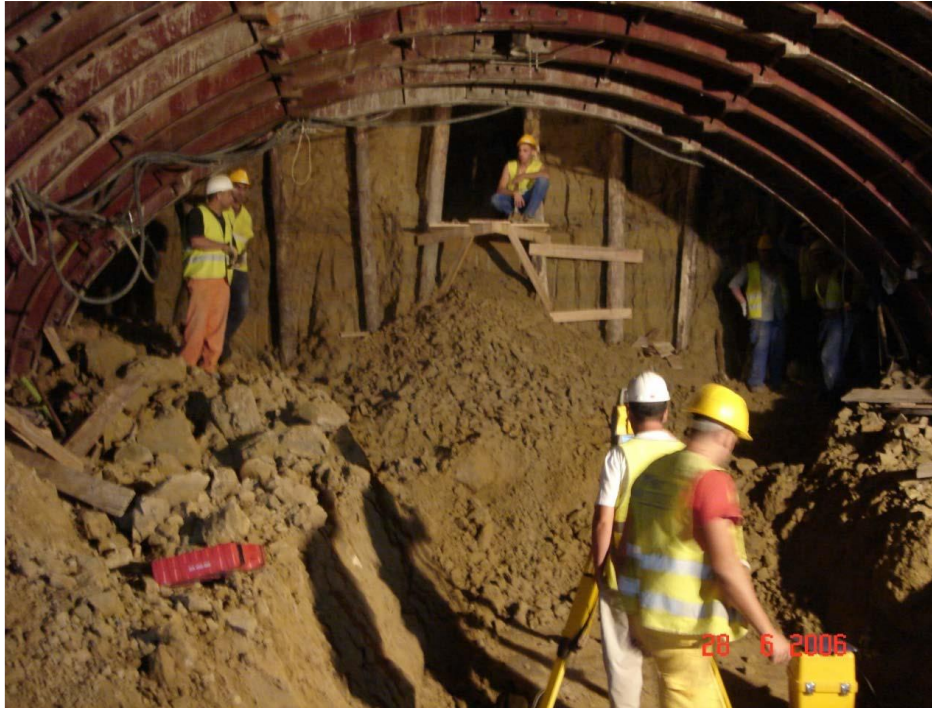
Figure 14 Excavation of a Gallery with Manual Methods (Professor García Menéndez, 2018)
