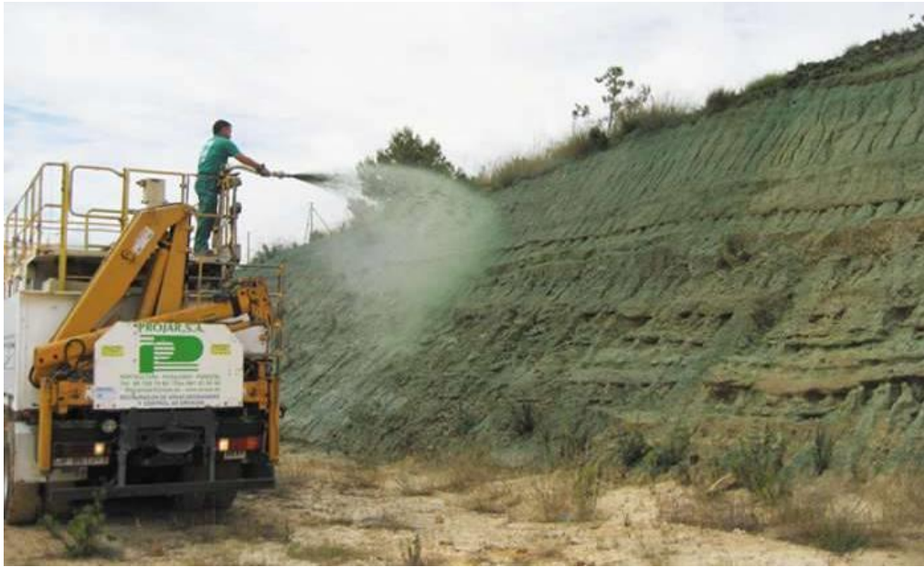
Fig 50. Hydro seeding technique
