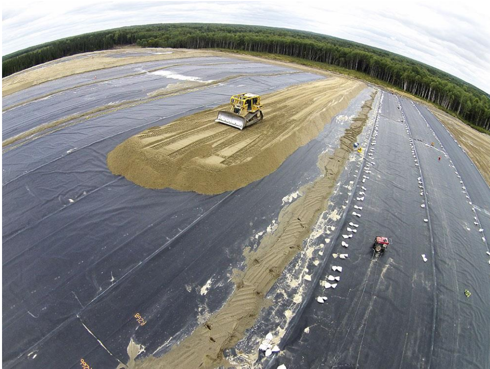
Fig 17. Geomembrane application in Barvue
