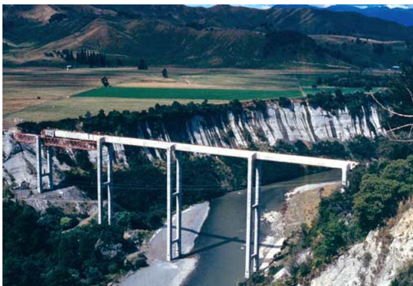
Figure 1.3: The South Rangitikei Railway Bridge.
