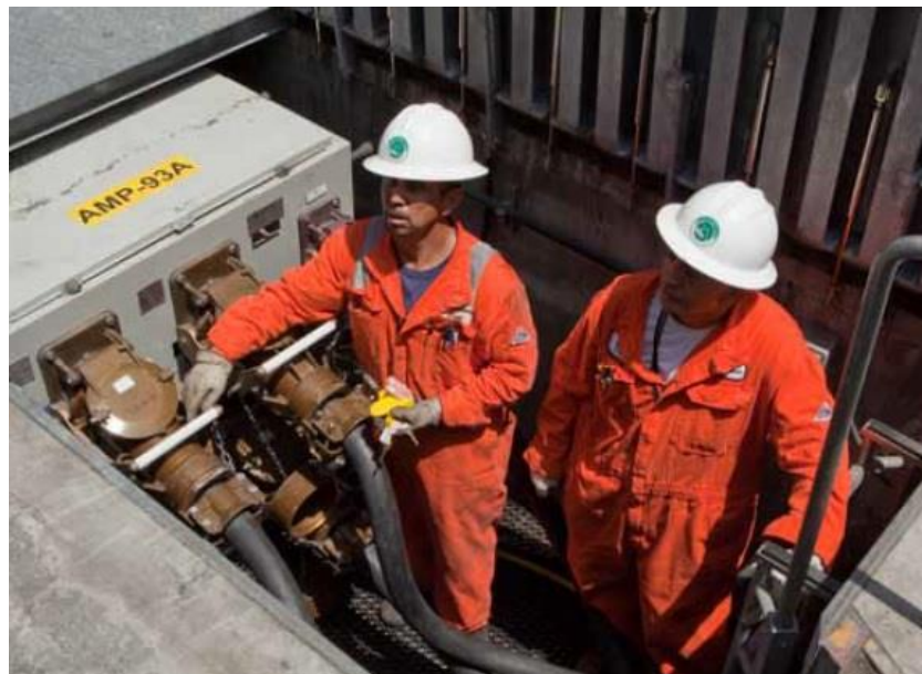
Figure 2.15 – Dual socket connection box inside the receptacle pit under connection process
