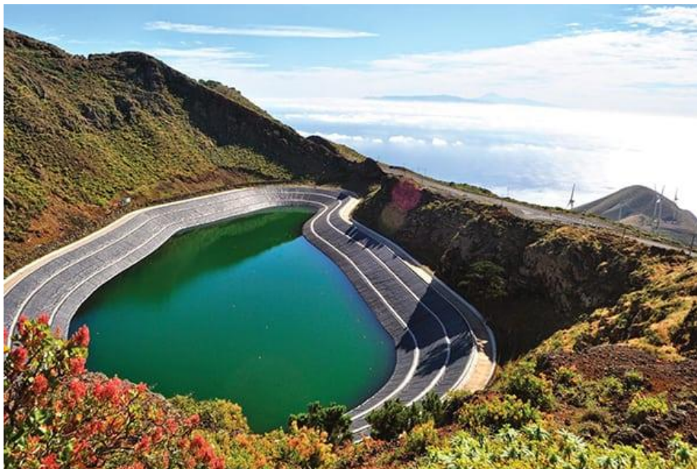
FIGURE 13: UPPER RESERVOIR OF THE PUMPED STORAGE SYSTEM
