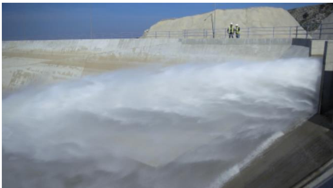
FIGURE 32: HIGHLIGHT DURING WATER PUMPING INTO THE ANO PROSPERA TANK
