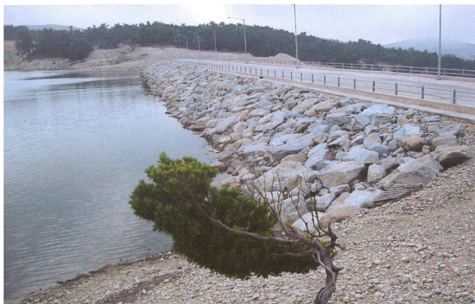
FIGURE 23: PEZI DAM (SOURCE: PPC SA)
