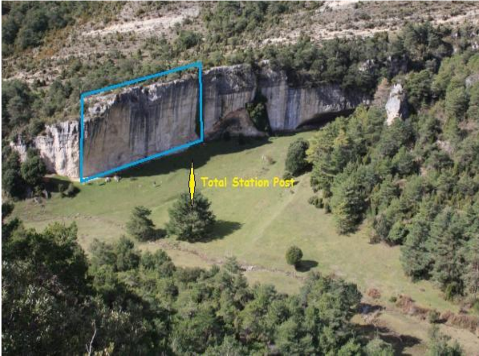
Image 2.3 Total Station set up station
