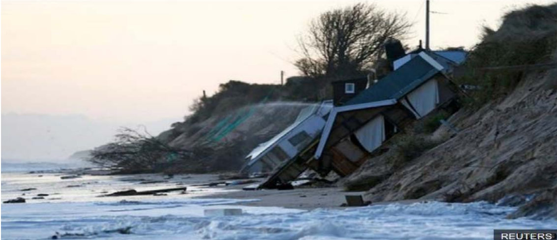
Εικόνα 3-12: Hemsby, on the Norfolk coast, UK (05.12.2013). «Seven cliff-top homes collapsed on the night of the worst storm surge for 60 years» [ www.bbc.com ]
