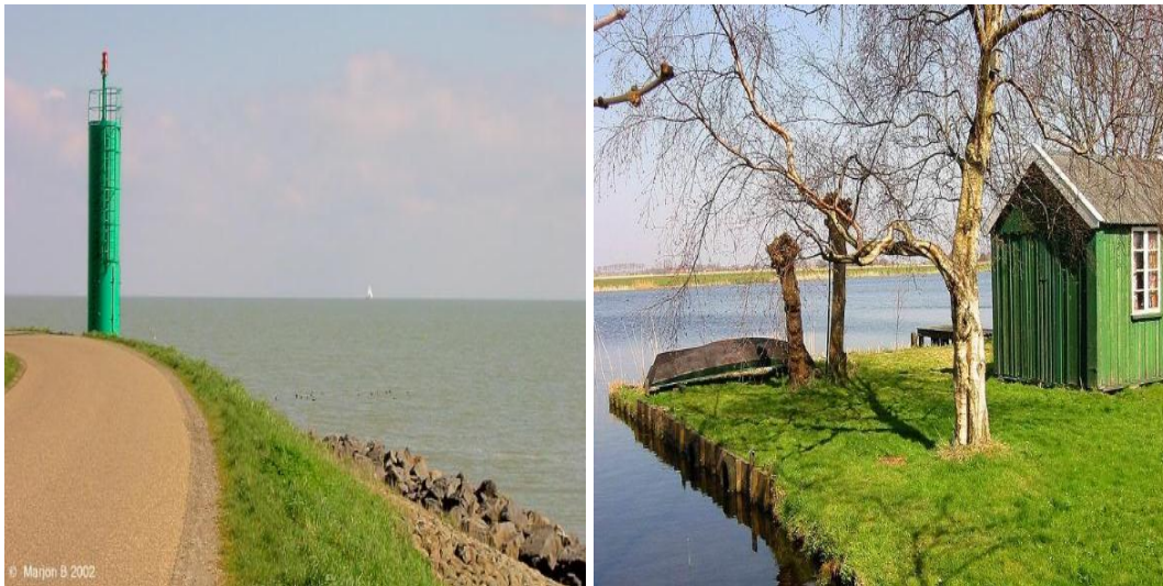
Figure 2.2: Dykes in Netherlands Source: Marjonnabar, Holland-Behind the Dykes, Webshot Channel, 2002
