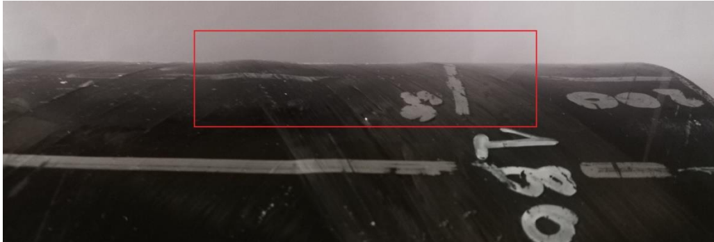
Figure 4.16 Uneven surface at 200 degrees, 50mm.
