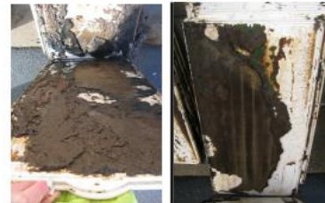
Photograph 3: Examples of severe sludge caking observed
