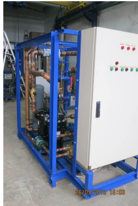
Figure 3.38 The finalized ORC engine and the modified expanders
