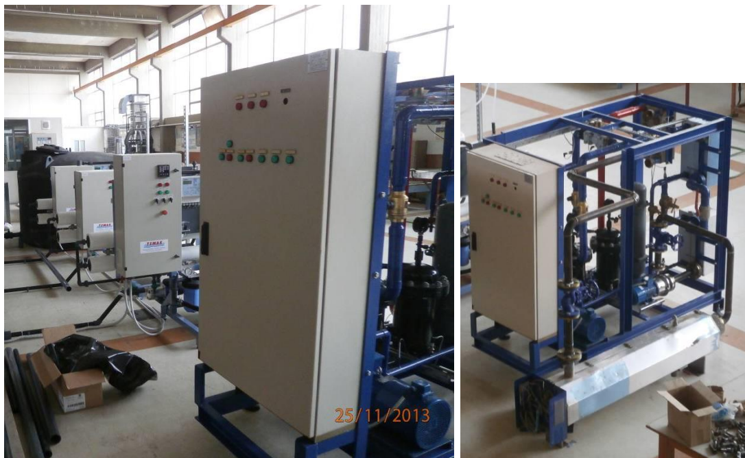
Figure 3.39 The ORC engine and the electric heater connection on the heat source cycle pump
