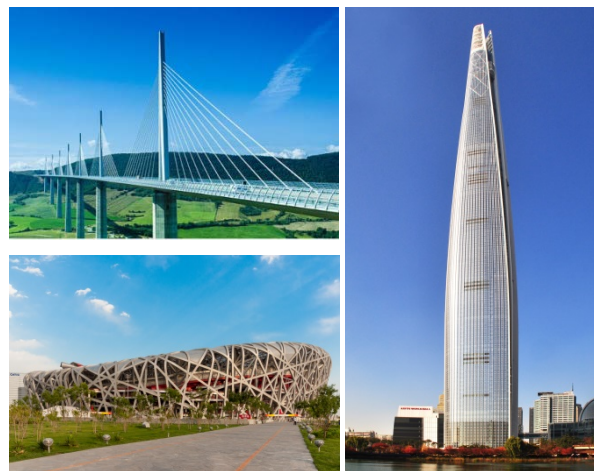
Fig. 2.6 Structural applications of HSS (Millau viaduct, Chinese National Stadium, Lotte World Tower)
