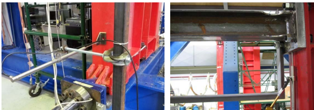
Fig. 3.9 LVDTs for measuring horizontal displacements of FUSEIS system and plate slippage
