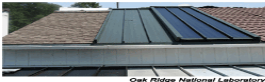
Three test roof assemblies at Oak Ridge National Laboratory: From left, shingle roof, metal roof with infrared-reflective (IR) coating, and phase change material/photovoltaic/metal roof.
