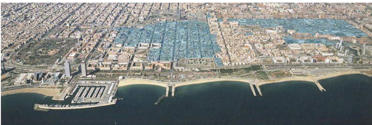
Εικ. | 4.2 22@ District. Πηγή: Barcelona: City, Architecture, Society, pg. 139
