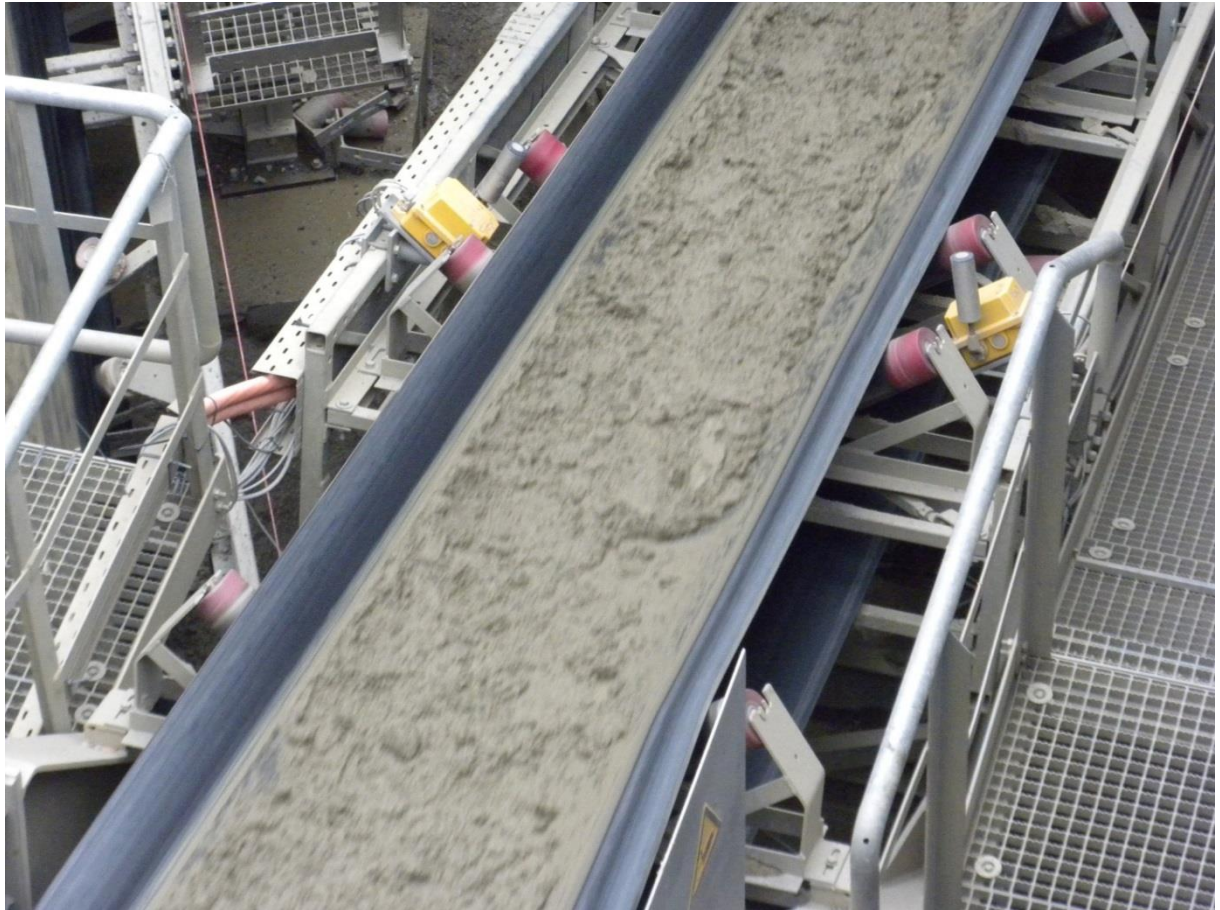
Figure 71: Field observation of EPB's conveyor belt of Athens Metro Line 3 Extension Project at Ag. Varvara Station (2).
