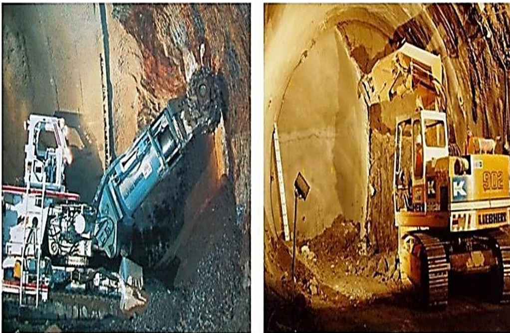
Σχήμα 2.1.β: Φρέζα(Roadheader)-Jersey, Exchange Place Station,2002(Sauer G.)
