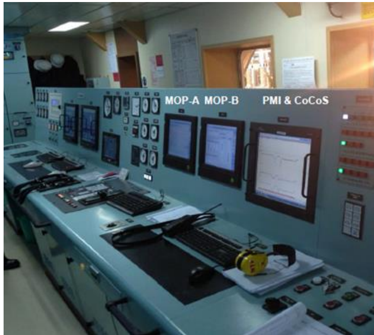
Figure 6.2: Engine Control Room Console [21]
