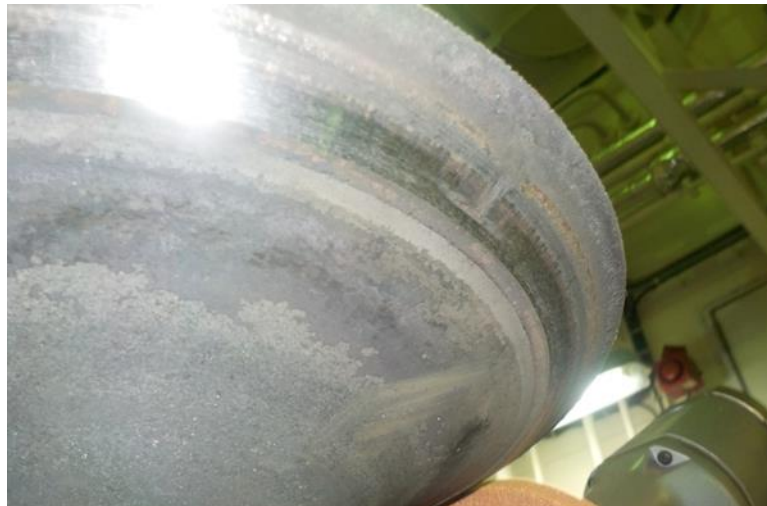
Figure 38: Photo of damage on exhaust valve spindle of Cylinder No.2
