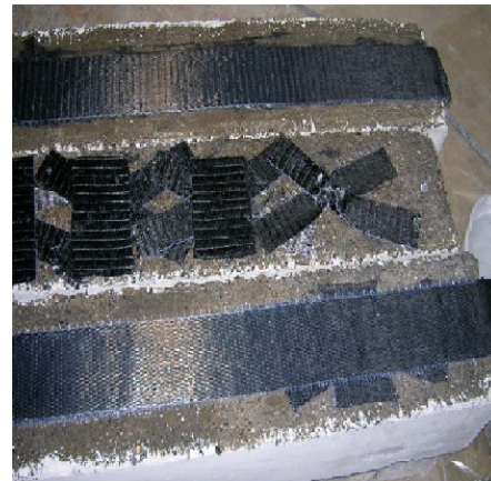
Figure 5: Placing of anchors & FRP application
