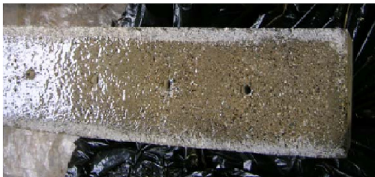
Figure 4: Drilling & placing of anchors
