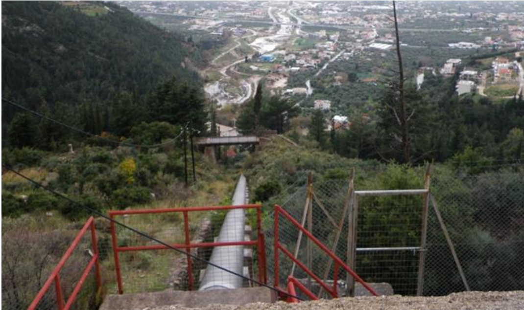
Figure 8.4: View of the penstock (Evaggelatos, 2016).
