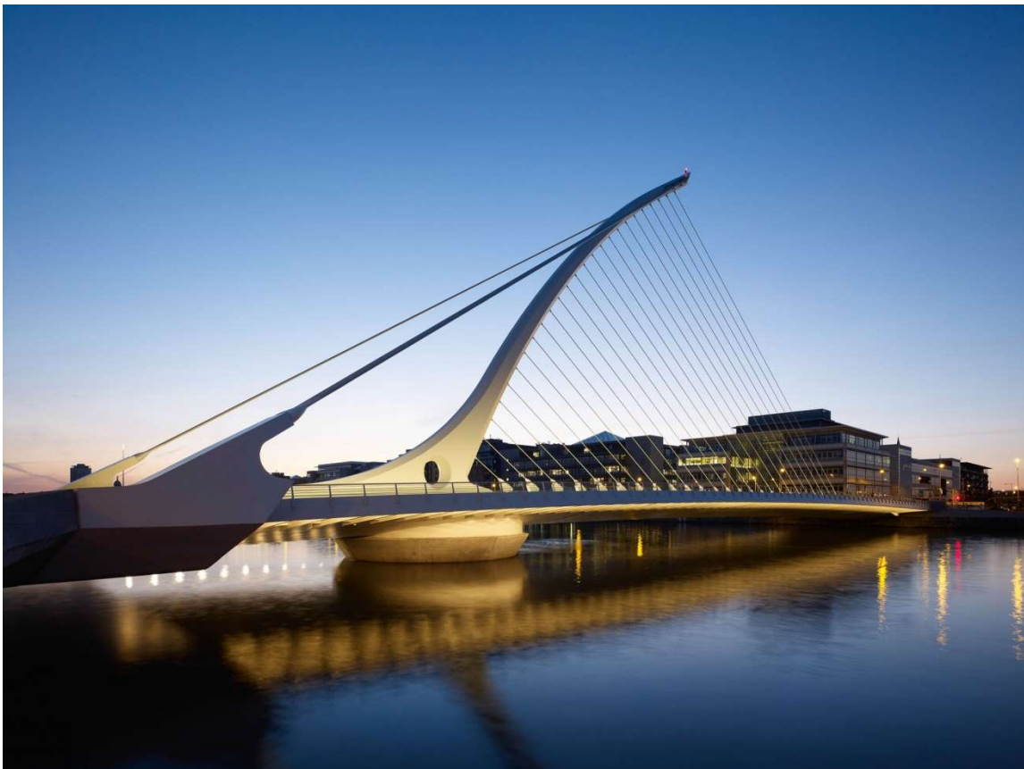
Σχήμα 1.1: Samuel Beckett Bridge, Santiago Calatrava, Dublin 2009
