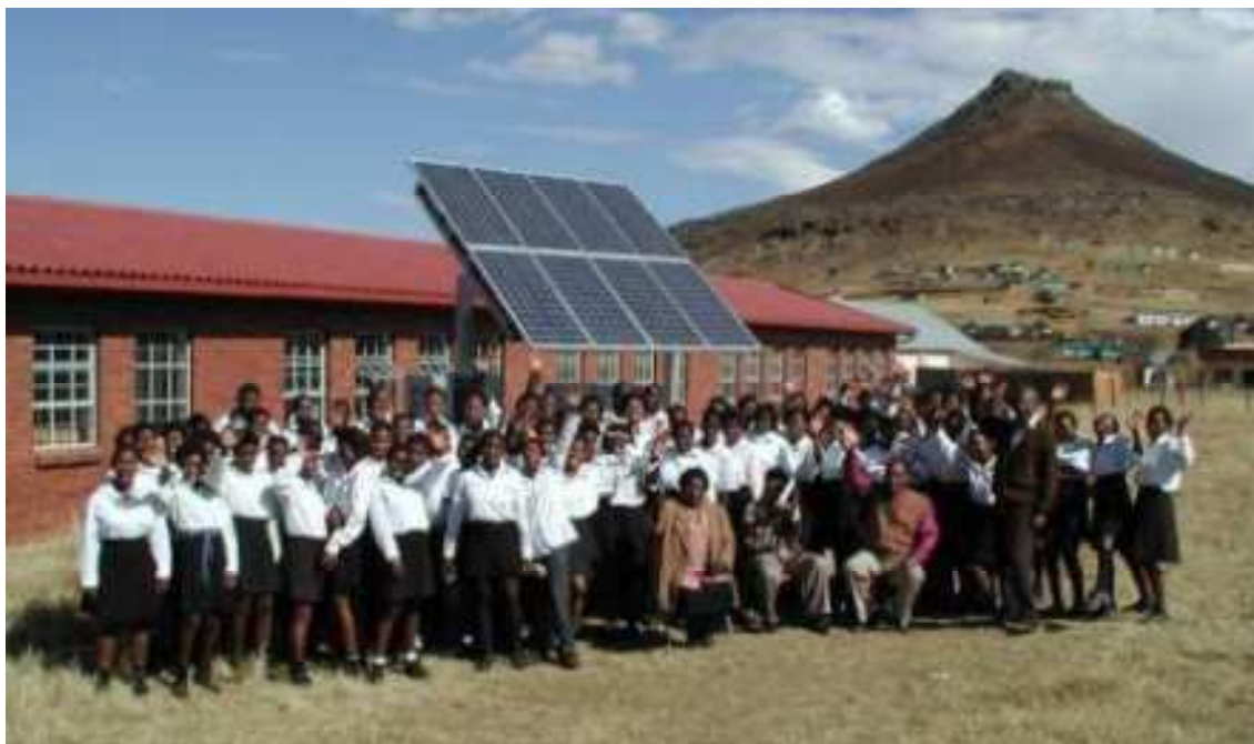
School in South Africa powered by a photovoltaic system
