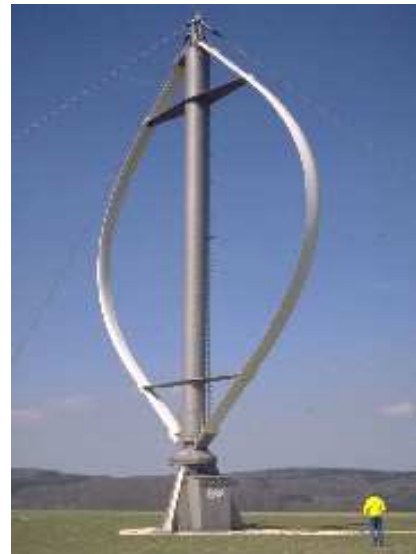
Darrieus wind turbine
