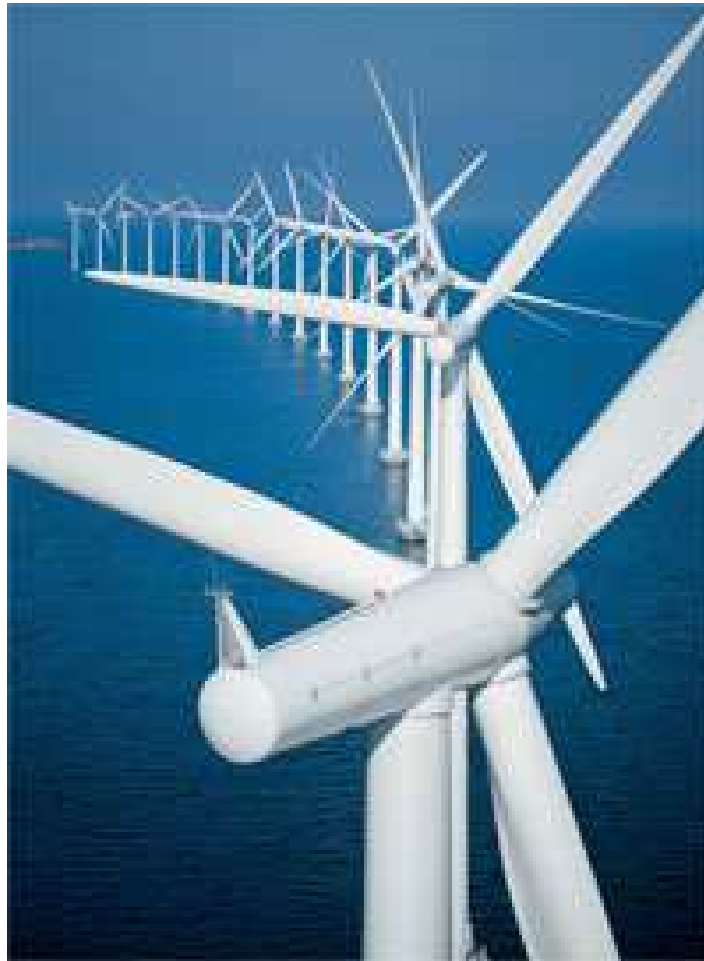
The offshore wind farm Middelgrunden near Copenhagen with 20 large 2MW wind turbines (total length 3,4 km)
