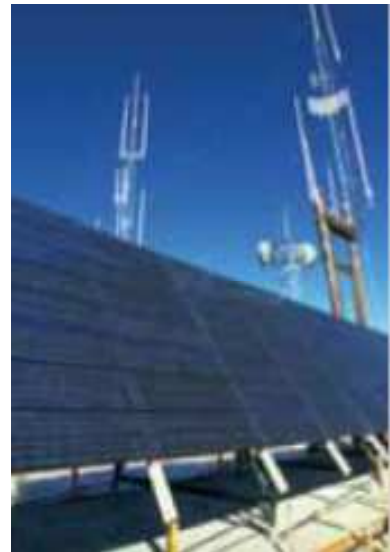
PV used for a remote telecommunication station
