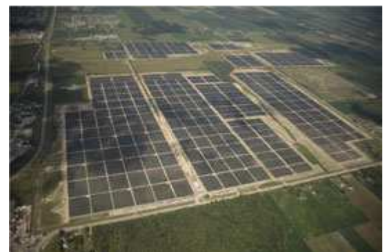
Sarnia PV power plant in Canada (97MWp)
