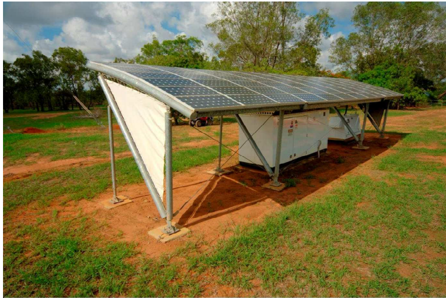
Solar-diesel hybrid station
