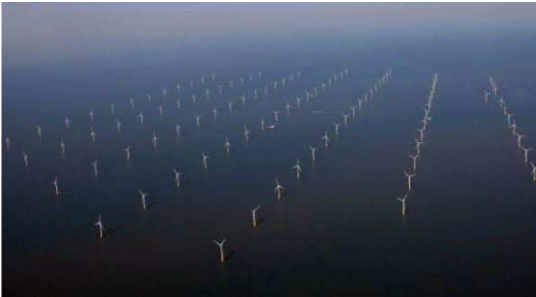
Aerial view of a wind farm located in the English Channel with 100 wind turbines of 300MW total capacity (area covered: 35km 2 )
