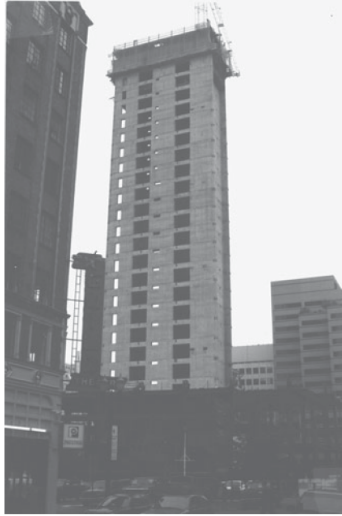
Fig. 2. Wall assembly in a building under construction
