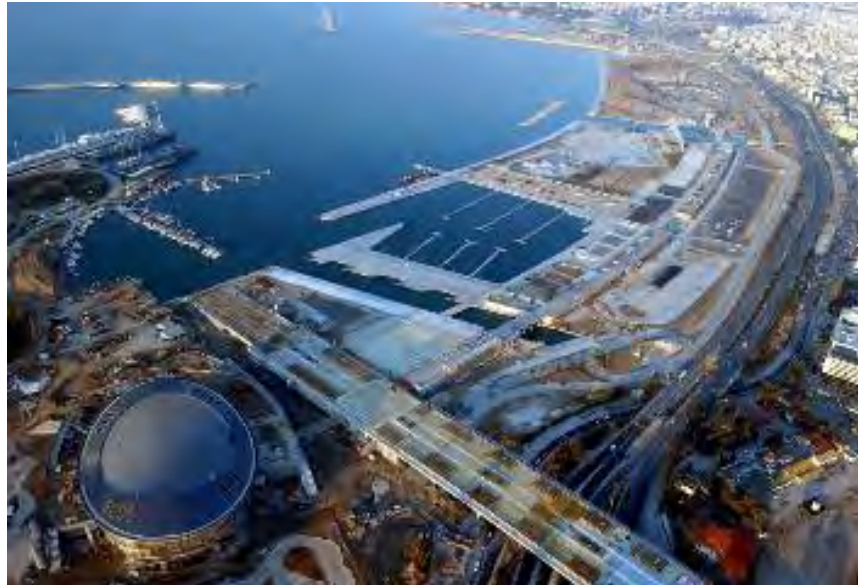
Faliron Bay: the massive construction of the Tae Kwo Do stadium (source: www.palaiofaliro.gr )
