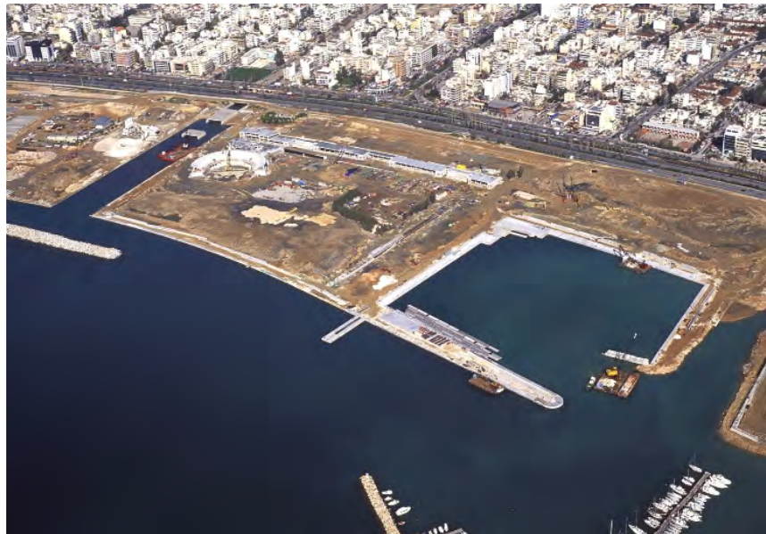
Faliron Bay during the construction of the Olympic Stadiums (source: www.palaiofaliro.gr )
