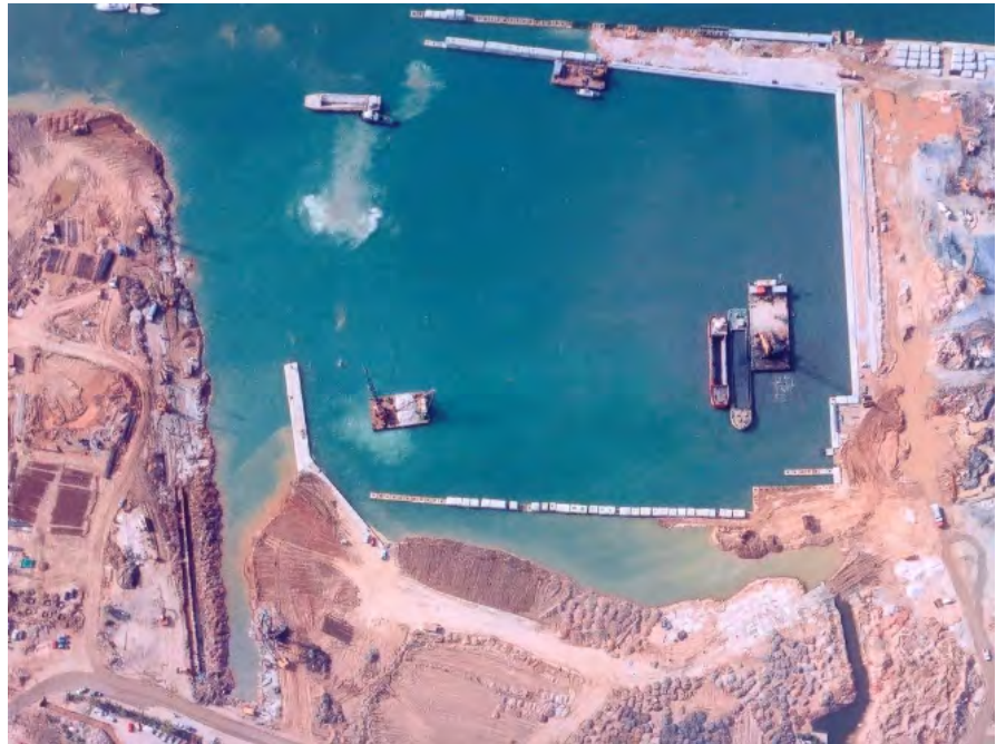
The formation of a new coast line and the embanking of the bay
