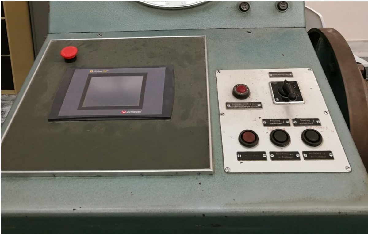
Figure 2.6: Control panel at fixed end
