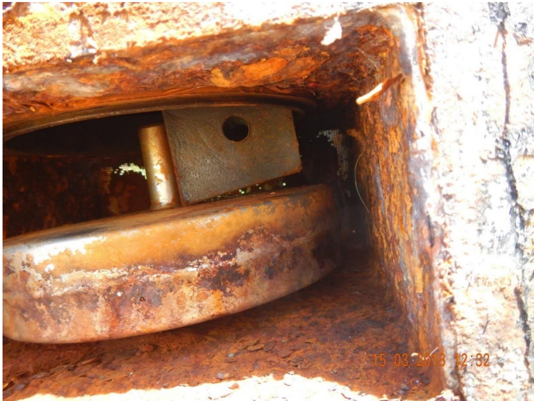
Figure 1.3: Instance of Corrosion in Water Ballast Tank Air Vent
