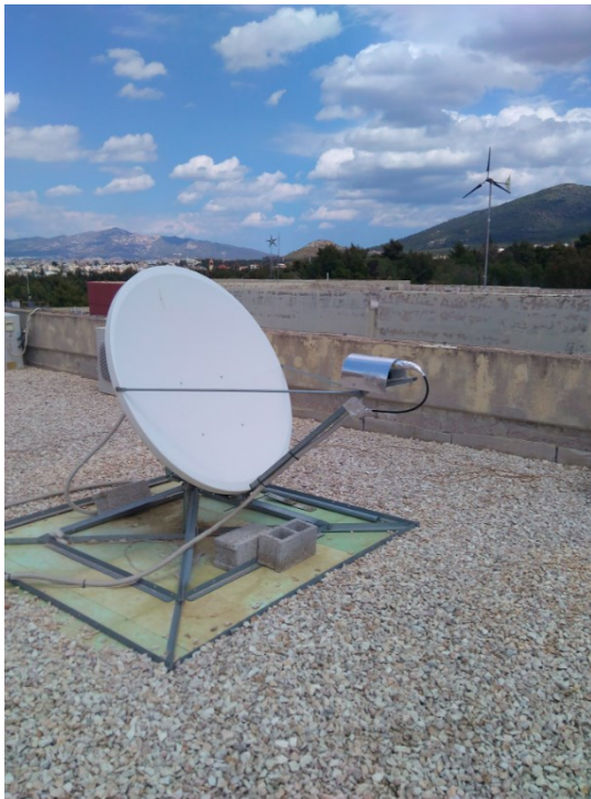
Figure 4-39: Front view of the antenna with the acrylic sheet installed around the LNB and feeder
