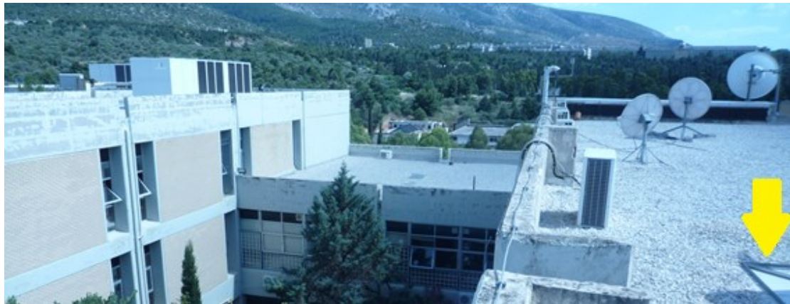
Figure 4-2: The deployment site at the NTUA Campus location.
