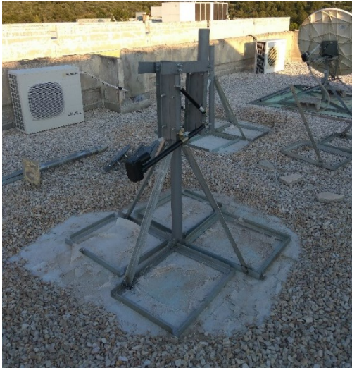
Figure 4-23: The finished Q-band antenna mounts
