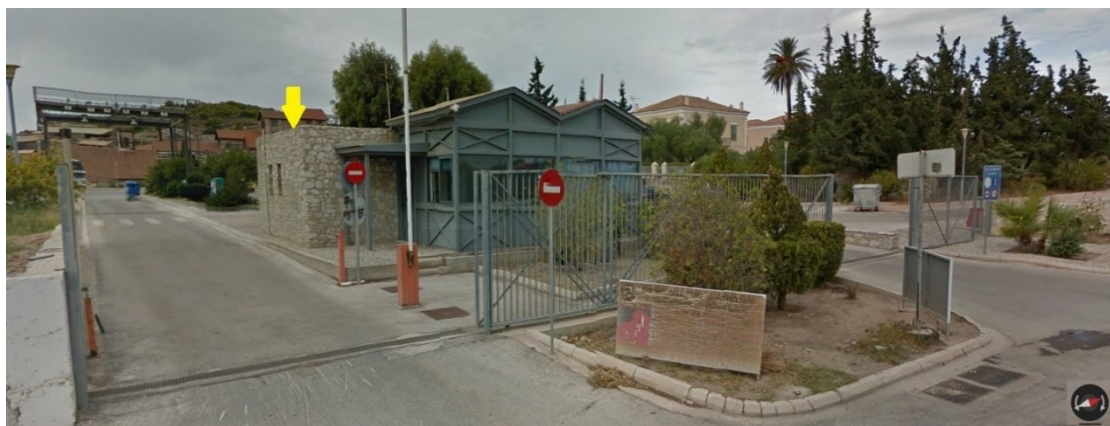
Figure 4-3: The deployment site at the NTUA LTCP location.
