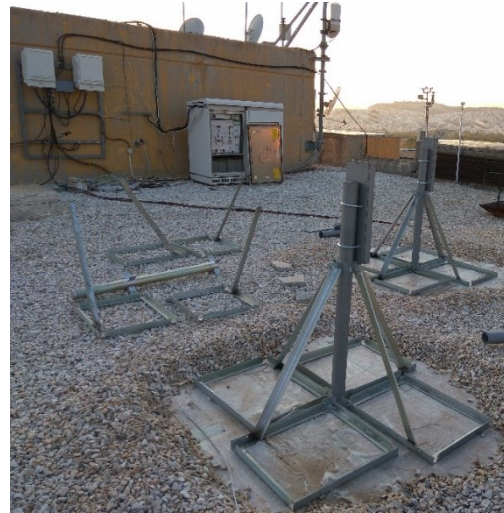
Figure 4-23: The finished Q-band antenna mounts
