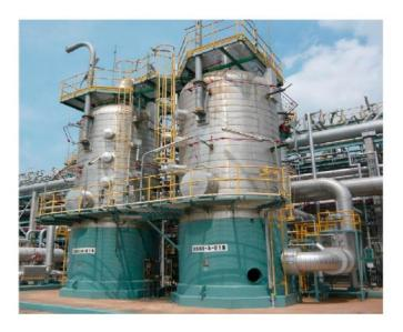
Figure 3.4. Parallel mercury removal units (fixed-bed reactors) at a Thai gas plant [10].
