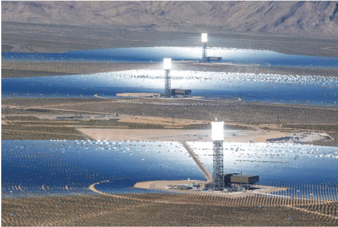
Figure 1-14. The Ivanpah Solar Electric Generating System [20]
