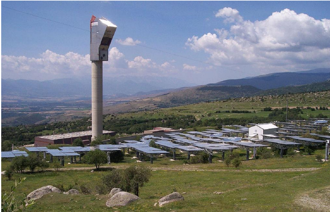
Figure 1-8. The Themis Solar Power Tower in the Eastern Pyrenees, France (Patel & Choksi, 2015) [15]
