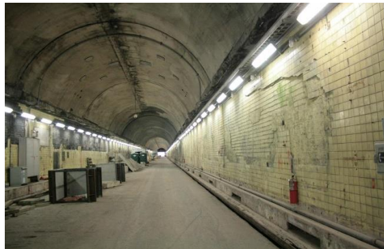
Figure 5.17. Overview of the multiple geometric features along the walls of the Memorial Tunnel, which constitute roughness elements.
