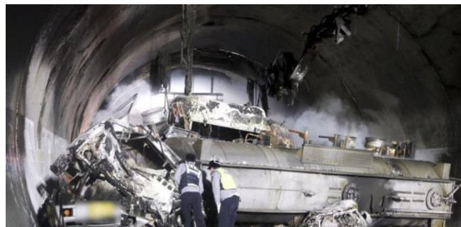
Figure 5.4. Three people lost their lives and other forty-three were injured in multiple expressway pileups, at Samae Tunnel fire, 2020.
