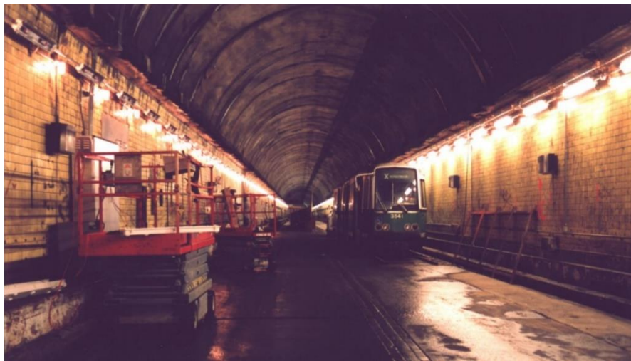
Figure 5.2. Internal view of the Memorial Tunnel, illustrating the cross-sectional geometry of the tunnel's configuration.
