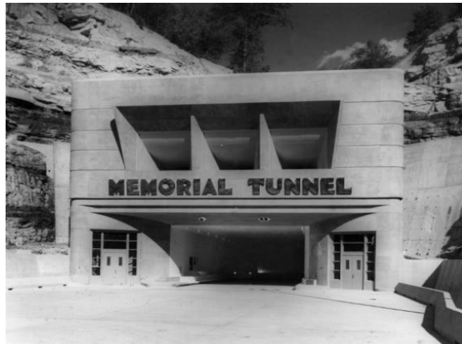
Figure 5.1. View of the north portal area of the Memorial Tunnel located near Charleston, West Virginia. ( https://transportation.wv.gov/Turnpike/about/turnpike_history/Pages/default.aspx )
