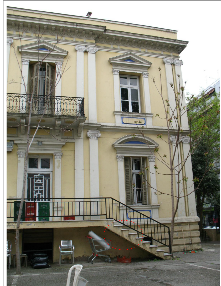
Description: Ph.10b- South part of west elevation.
