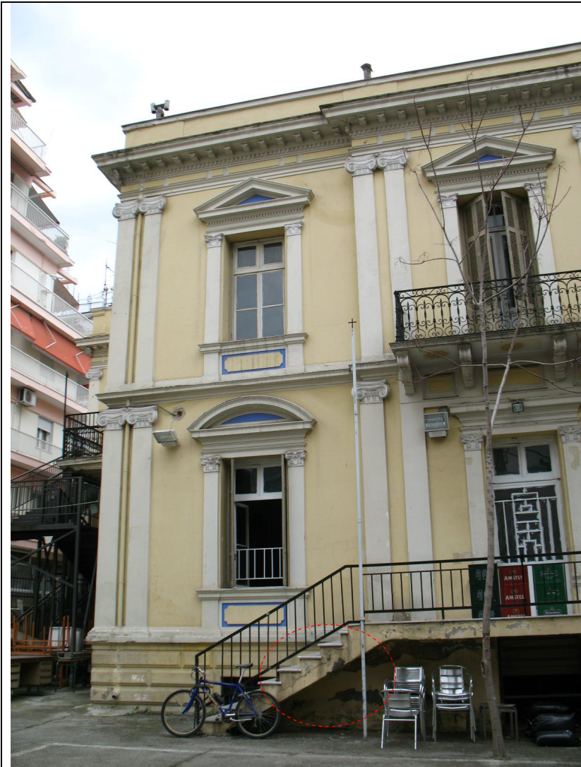
Description: Ph.10a- North part of west elevation.
