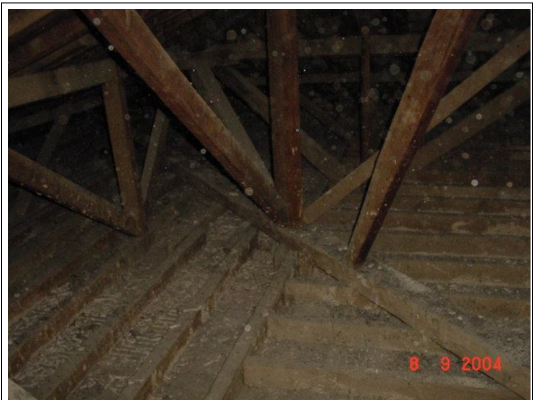
Description: Ph.47 – Another side view of similar elements, as per ph.46.
