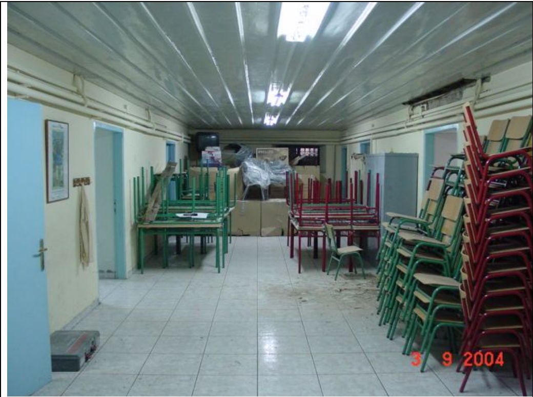
Description: Ph.70 – General view of Y1 at basement.
