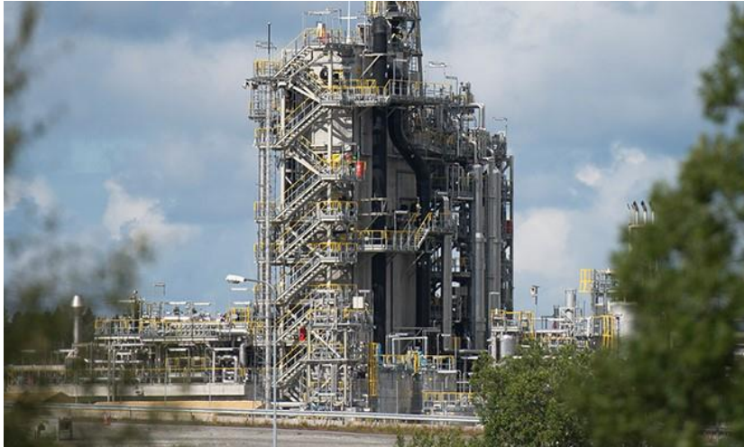
Figure 7: Post combustion Carbon Capture Liquid Solvent based tower (ten stories high building, equivalent to approximately 30m) [7]
