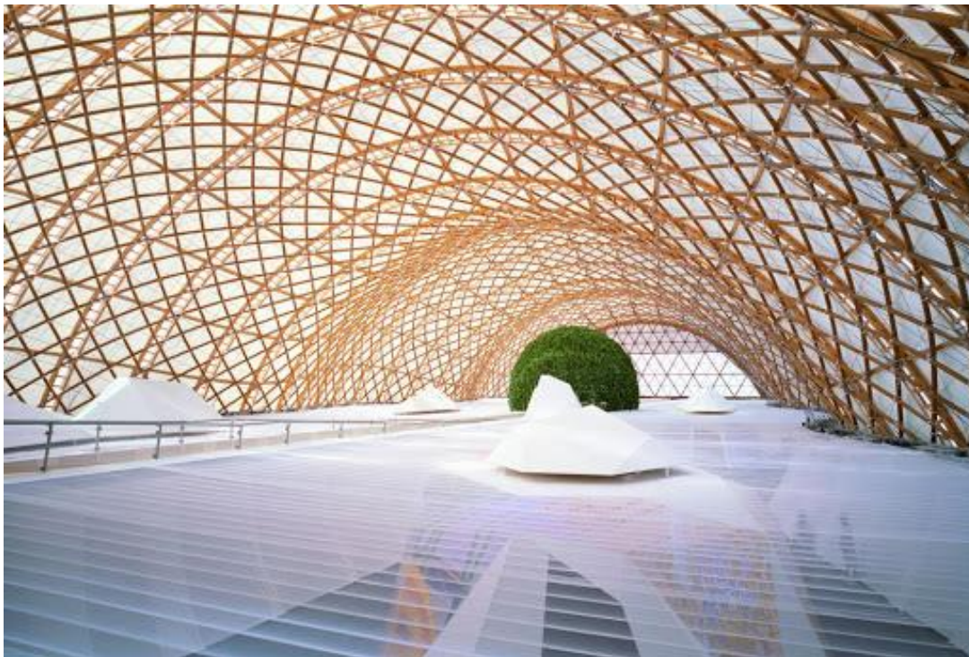
Figure 3.9 Timber gridshell, Japanese Pavilion (Expo 2000) by Shigeru Ban and Frei Otto, Hanover, 2000
