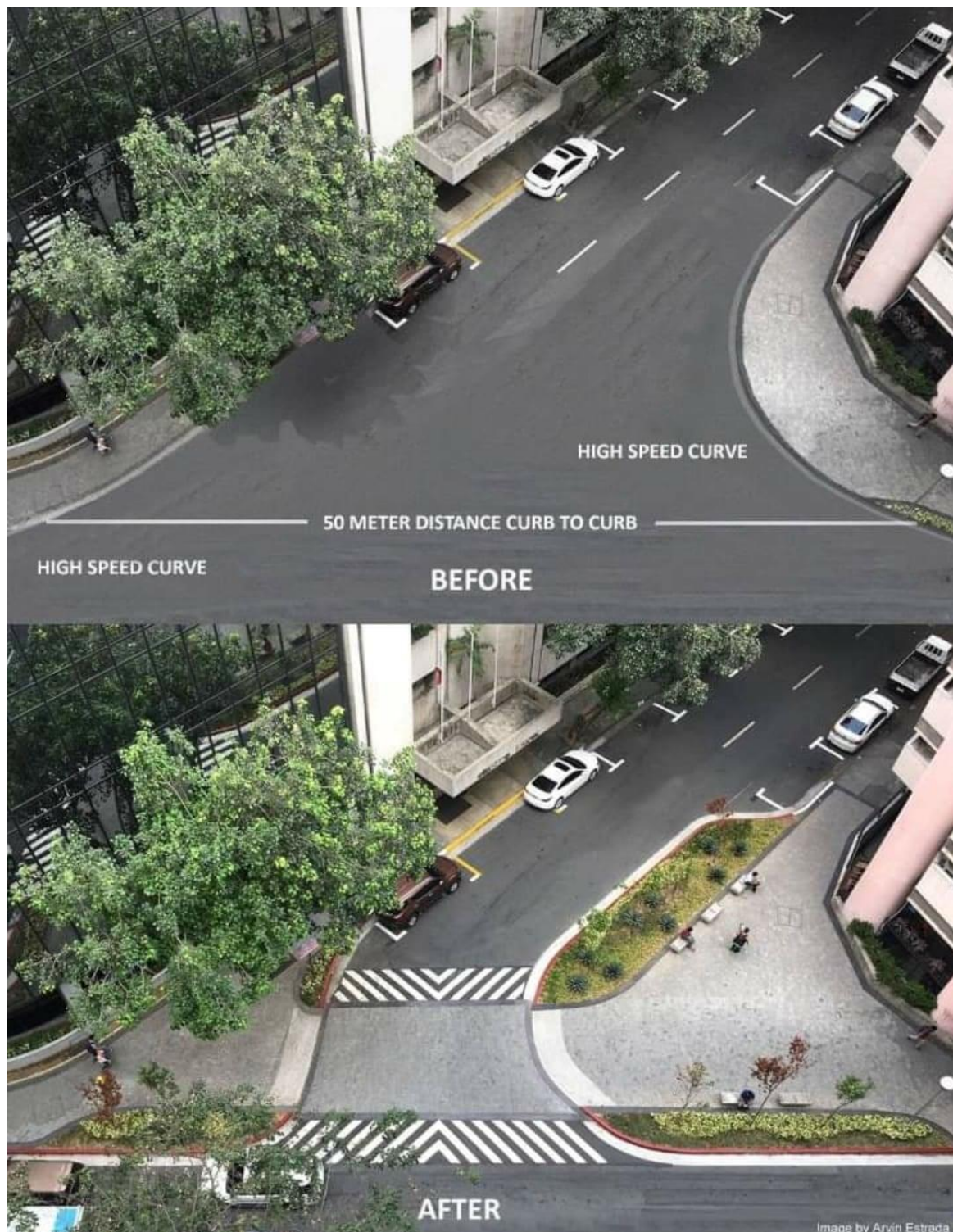
Figure 2.13: Changes in road architecture and design to pedestrian-friendly solutions
