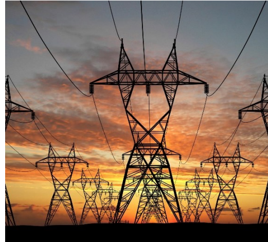
(b) Delta tower with one circuit
