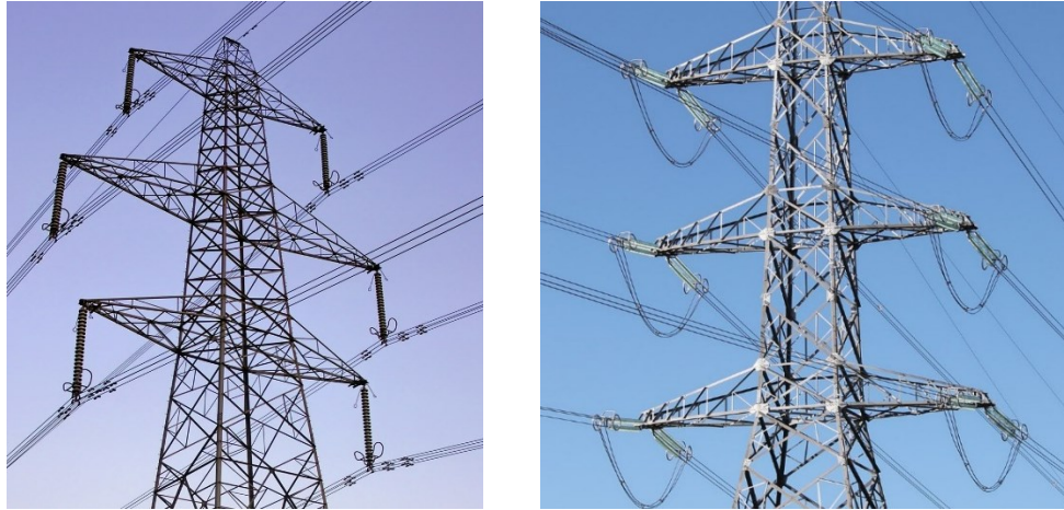
Figure 8.2: Suspension tower (left) and dead-end tower (right)
