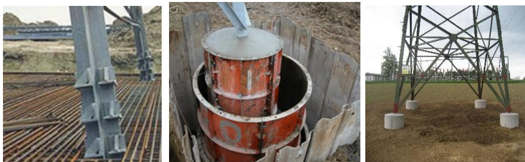
Figure 8.8: Step foundation of a lattice tower
