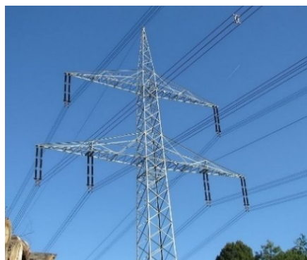
Figure 9.1: Danube tower for a transmission line of 380 kV
