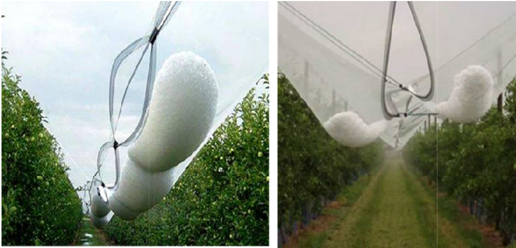
Figure 6.7 The deformed shape of the roof under the accumulated load
