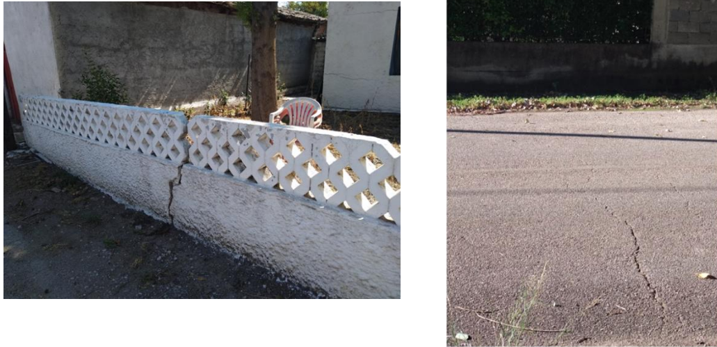
Figure 1: Damages to buildings and infrastructure at the study area.
