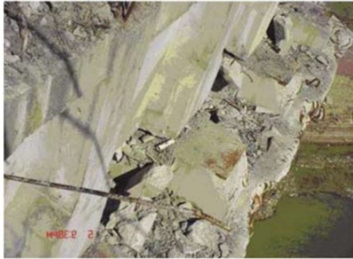
Figure 20 Span collapse of the Miaoziping Bridge
