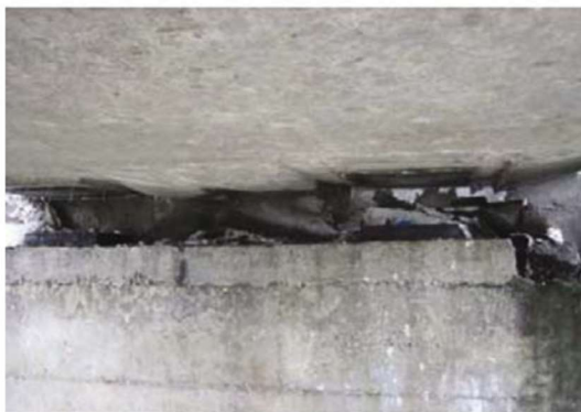
Figure 19 Huilan Bridge damage during Wenchuan earthquake
