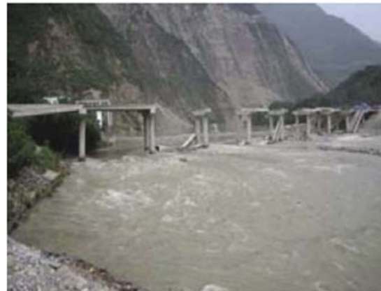
Figure 21 Girder failure for Gaoyuan Bridge and Nanba Bridge respectively.
