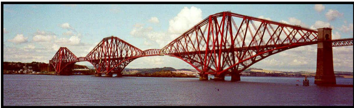
Σχ. 1.12. Γέφυρα Firth of Forth
